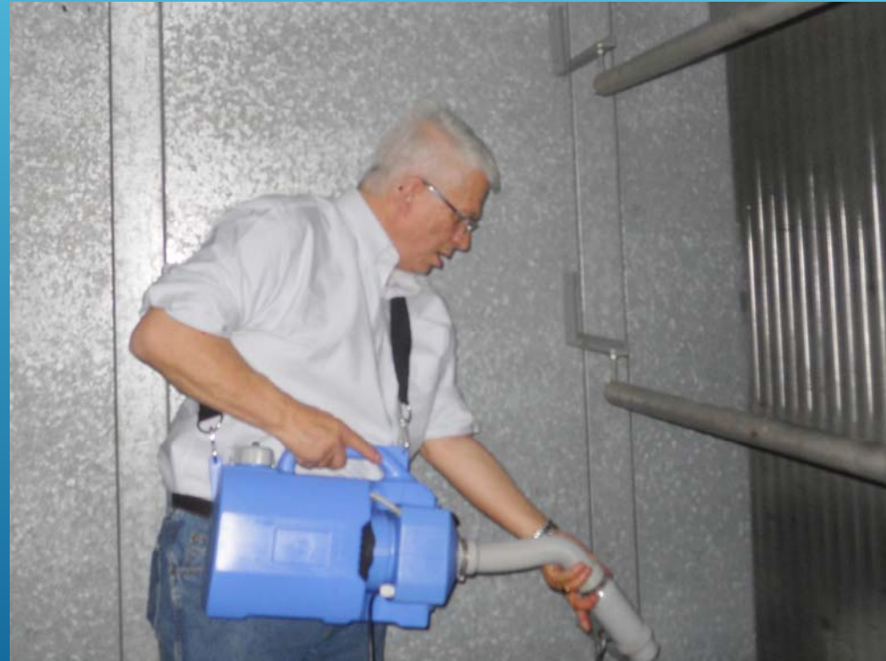
Fogging the cooling coil
