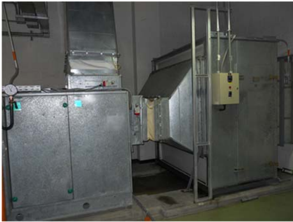
Typical Chilled Water HVAC AHU's
