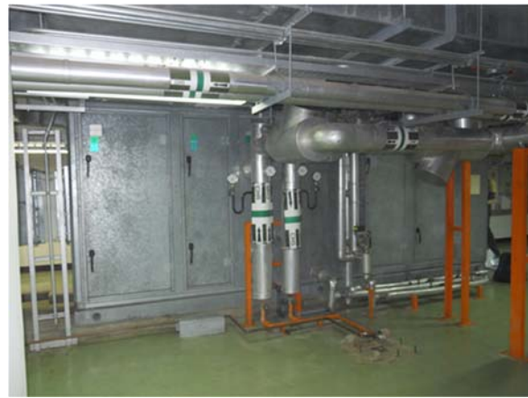
Typical Chilled Water HVAC AHU's
